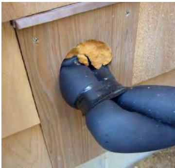
Envelope penetration not sealed properly Source: Marc R., Minisplit Heat Pump Lessons, South Mountain Company, Martha's Vineyard, MA
