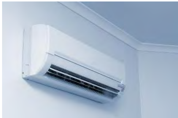
Indoor units located more than 30 cm below the ceiling (best practice 30-45 cm from ceiling) Source: www.pinterest.es
