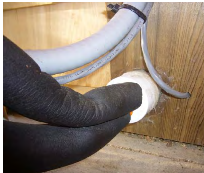
Envelope penetration properly sealed Source: Marc R., Minisplit Heat Pump Lessons, South Mountain Company, Martha's Vineyard, MA
